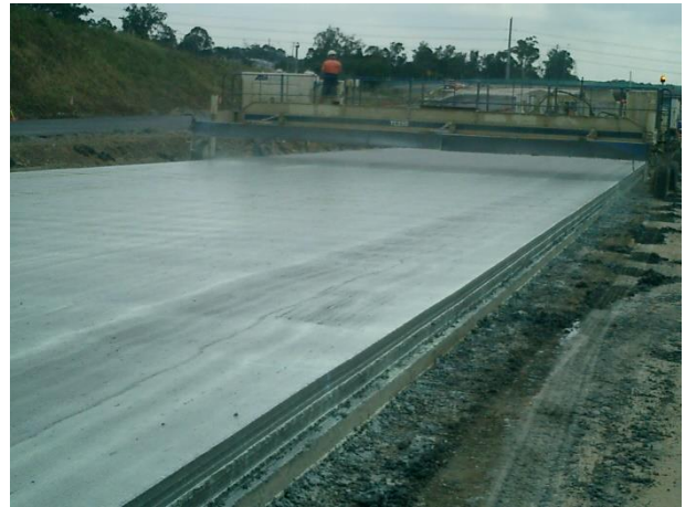
Surface Cure R being used on the M7 southwest Sydney
